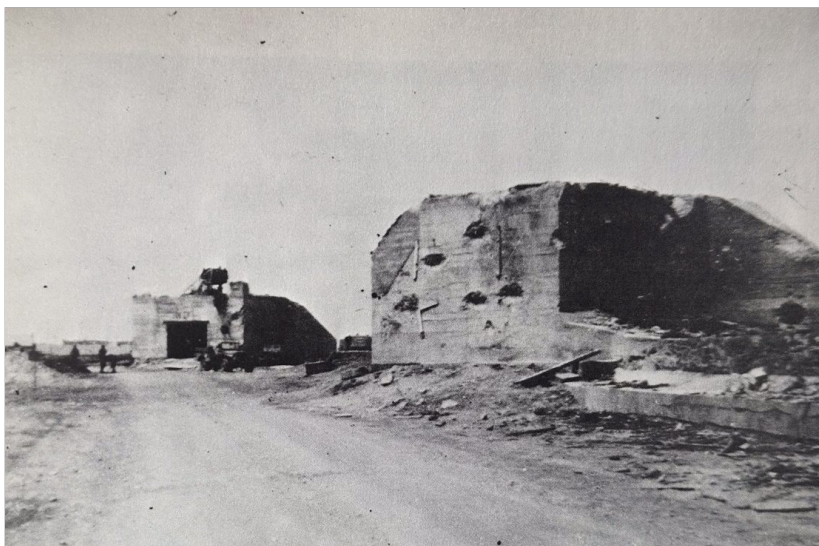
Huge German forts near Utah Beach show signs of battering from American big guns, probably naval. The blockhouses were visited by 535th troops after they had been neutralized. —Thomas P. Elliott photo
